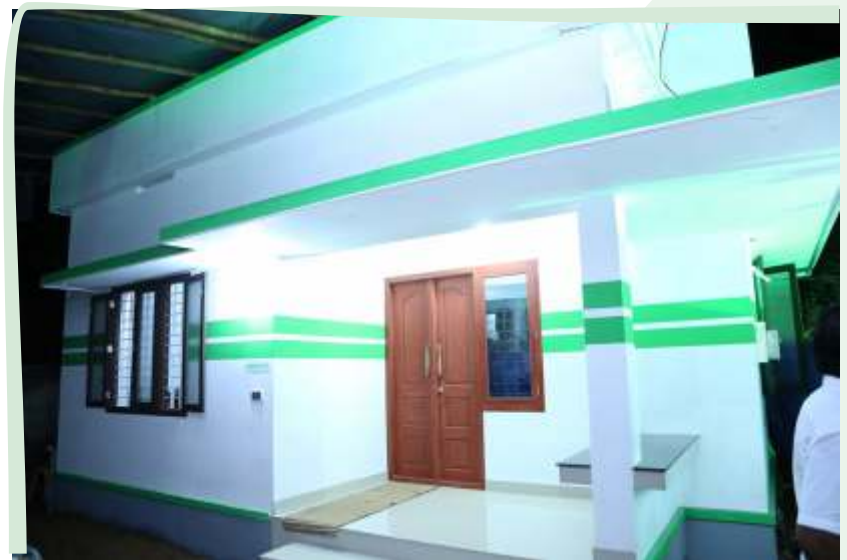
House after renovation and ready to handover
